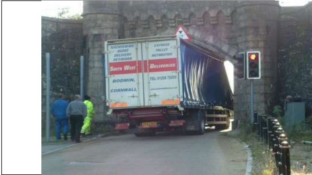
This Grade II Listed arch (by I.K.Brunel) was damaged again last year.
